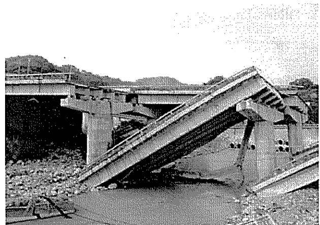
Photo 1. Bridge with Falling Spans
