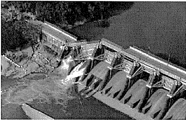
Photo 7. Shikung Dam after Earthquake
