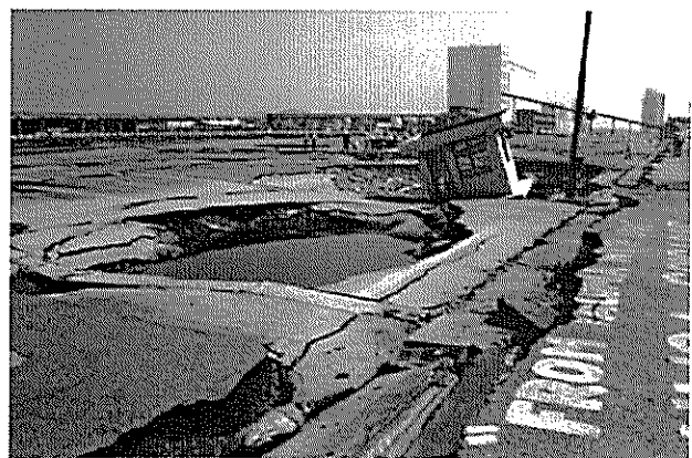
Photo 10. Damage to Taichung Port Due to Liquefaction
