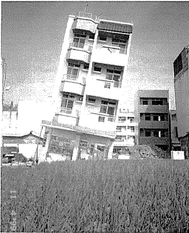
Photo 8. Foundation Failure Due to Liquefaction
