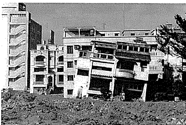
Photo 9. Building Damaged by Lateral Spreading
