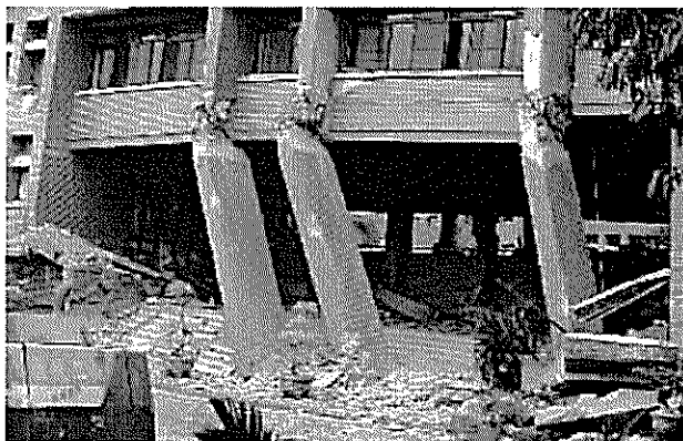
Photo 3. Building with Weak Ground Floor
