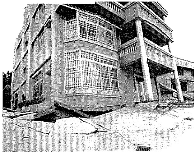
Photo 6. Building Damaged by Ground Movements
